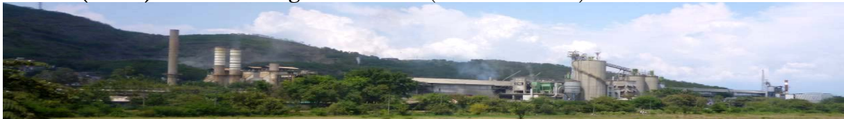
Abb. 23: Betonfabrik in Yumbo (CHRISTOPH 2012)
